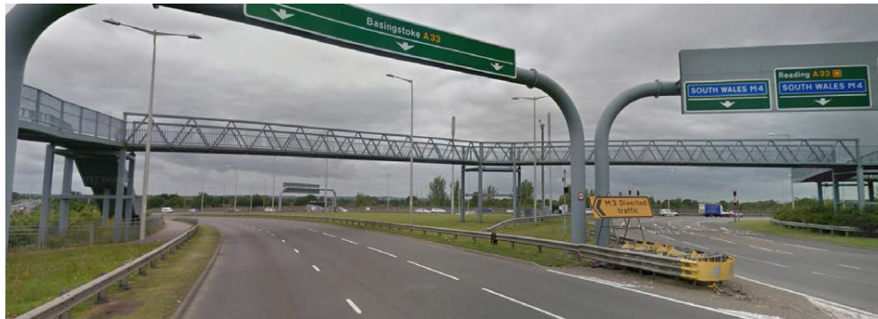
View of site with masts and lampposts to the South of Three Mile Cross Interchange
