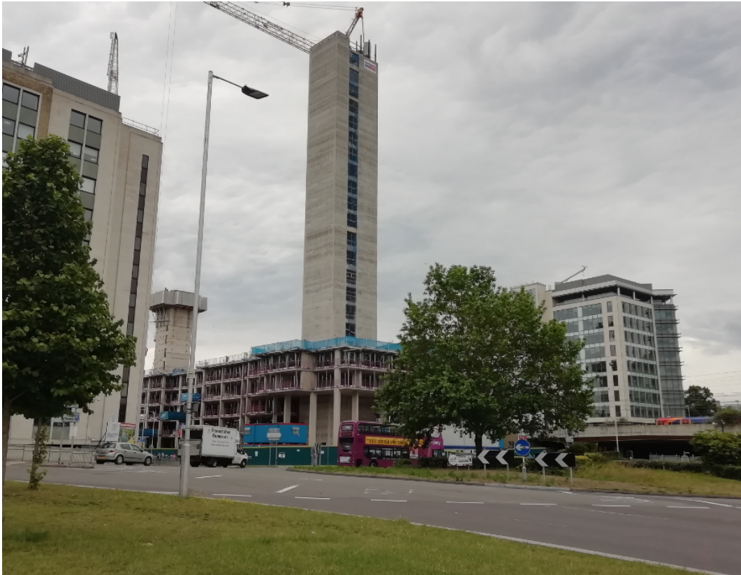
Photo 1: View southeast from Vastern Road roundabout (18 th June 2019 Conlon).
